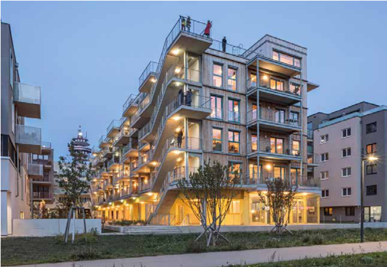
The ground floor of Gleis 21 is designed to be open and accessible to the public, housing a cultural center that includes a music school, a media studio, and an event hall.
