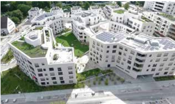
The certified passive houses are equipped with photovoltaic panels.
